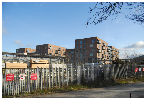
Western boundary of the Study Area with security fence forming the boundary, looking northeast (top)
